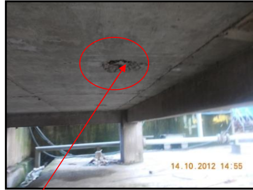
Segregation and spalling of concrete noted.
