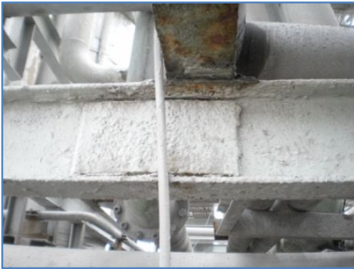
Severe corrosion
