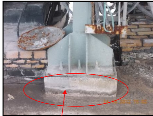
Seepage, moss growth & cracks at top finishing layer of pedestal.
