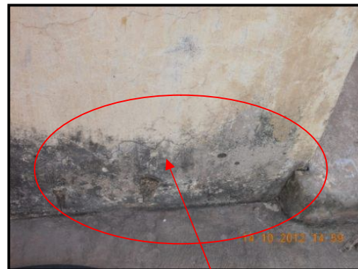
Cracks at the subsequent concrete pours & segregation noted .
