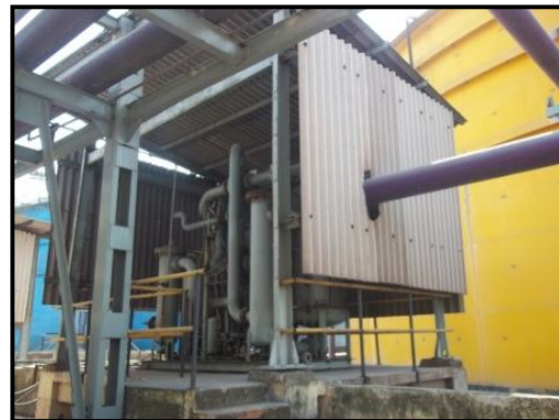
Corrosion and peeling of paint noted on the column.
