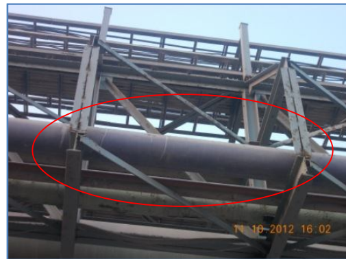
Corrosion, scaling and cut/slotted cross bracing
