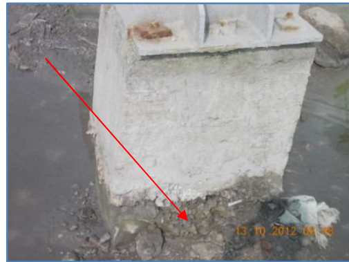
Scaling, corrosion on base plate and gusset plate also vegetation growth and honey combing
