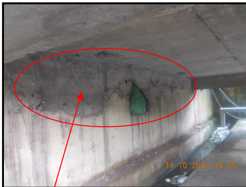
Cracks at the subsequent concrete pours & segregation noted .
