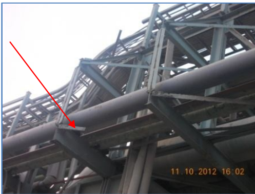
Corrosion, scaling and cut/slotted cross bracing
