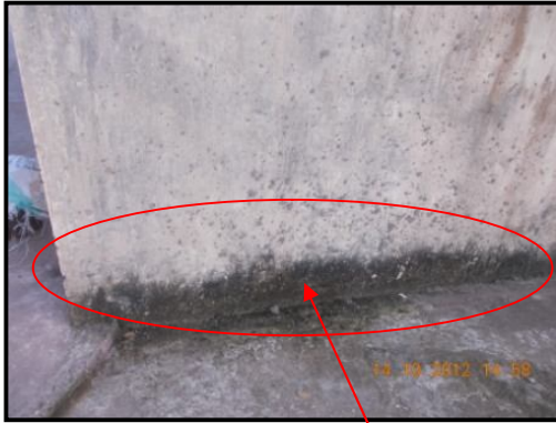
Segregation and spalling of concrete noted.
