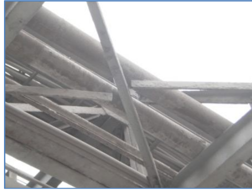
Inadequately welded connections
