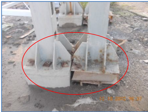
Scaling, corrosion on base plate and gusset plate also vegetation growth and honey combing
