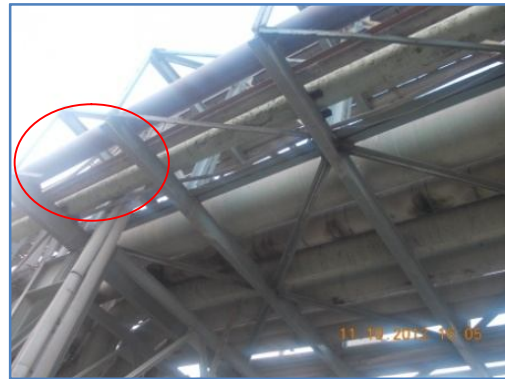
Cut/slotted cross bracing
