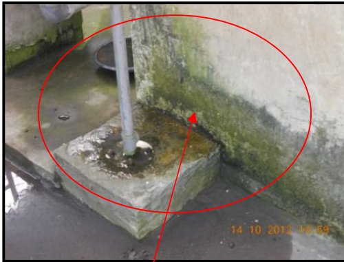
Seepage, moss growth & cracks at top finishing layer of pedestal.
