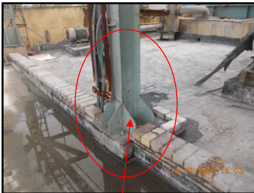
Corrosion and peeling of paint noted on the column.
